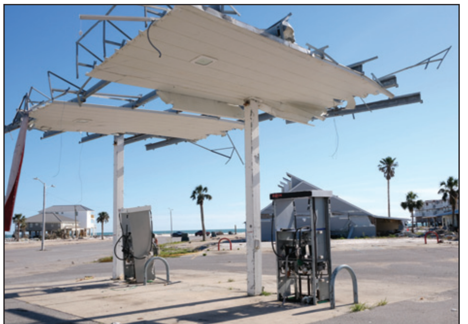
Mexico Beach has no gas station at the moment. This is one of three that were destroyed.
