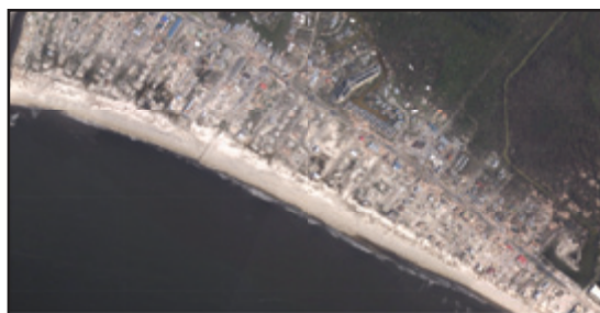
NOAA PHOTO Aerial view of catastrophic damage in Mexico Beach, Florida which suffered a direct hit from Hurricane Michael on Oct. 10, 2018.
