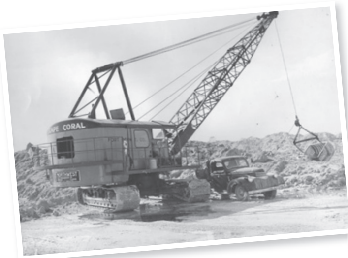
From left: Some of the heavy equipment used by workers hired by Cape Coral founders the Rosen brothers, to dredge canals. Their company, Gulf American Land Corp. (GAC), used the dirt for lots. Early Cape Coral seen from above. GAC salesman Ken Schwartz poses with dredging equipment. Cape Coral has 378 miles of canals.
