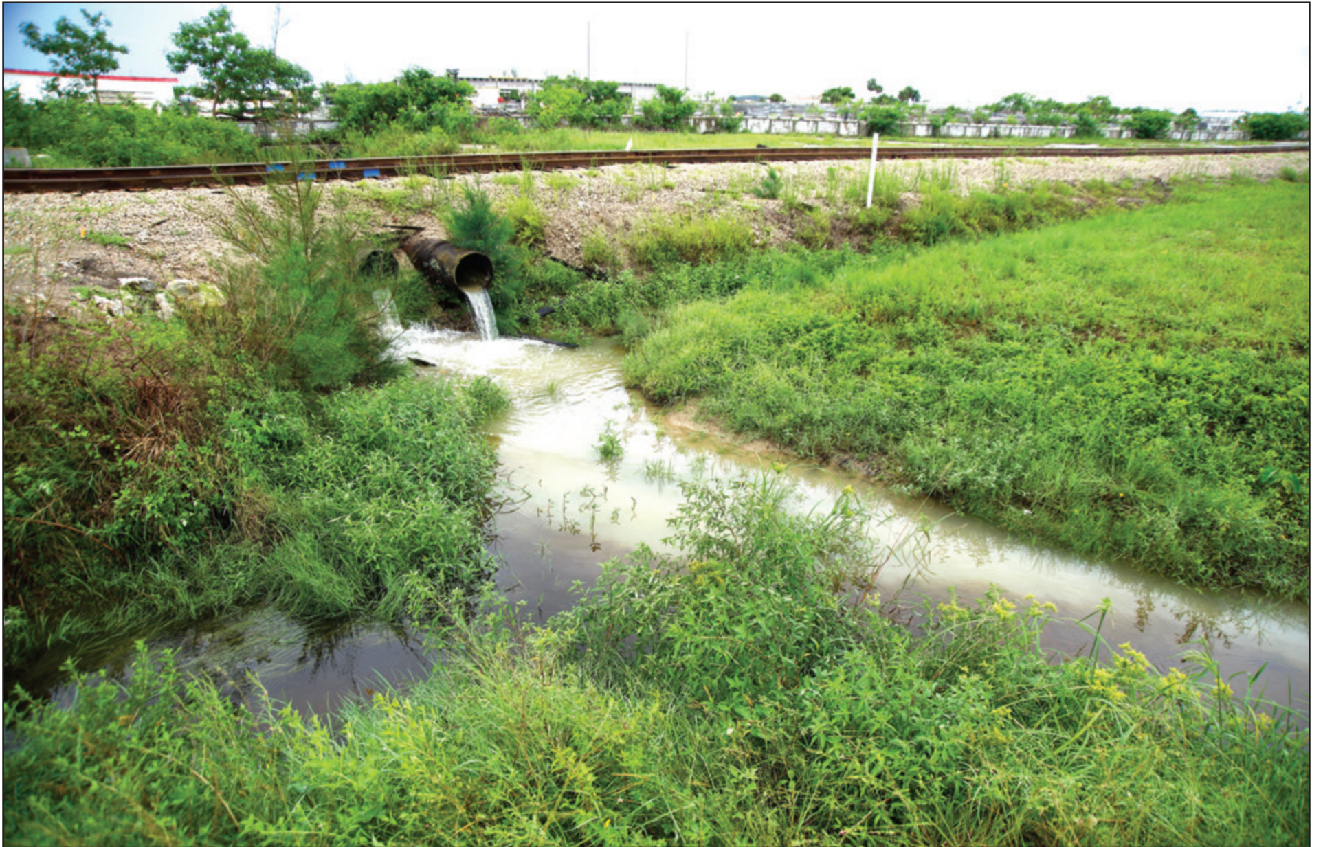
Manuel Branch Canal intersects with Ten Mile Canal just past the end of Canal Street in Fort Myers.
