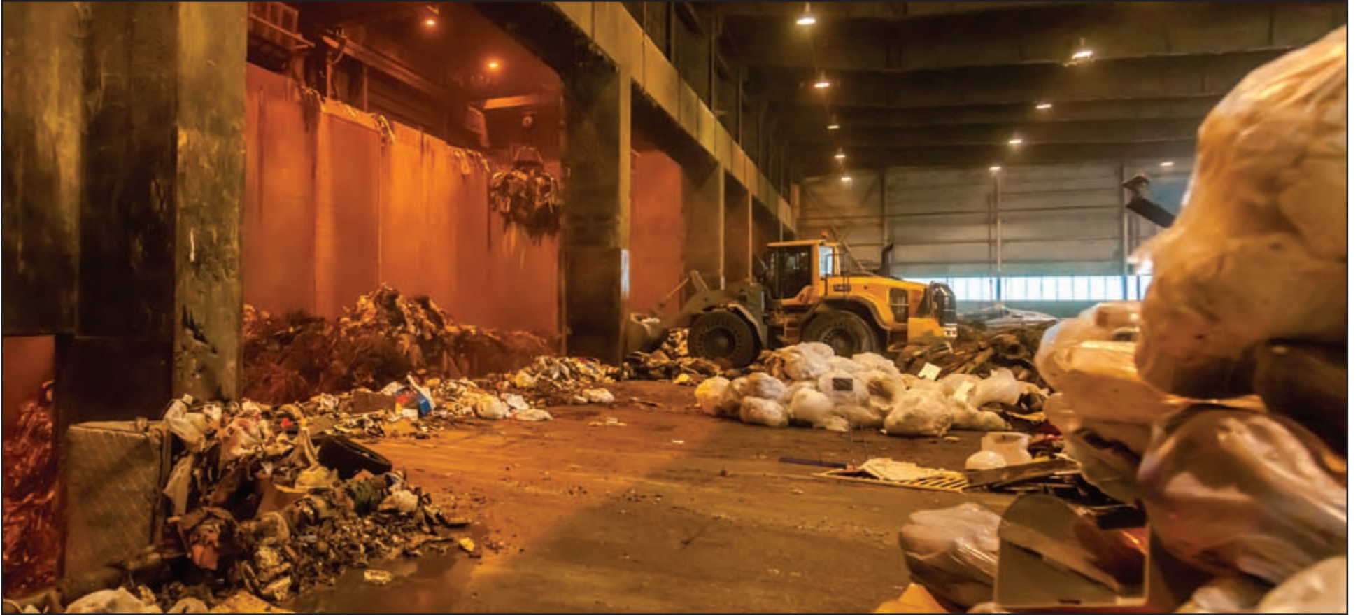
In Lee County, garbage is dumped onto the tipping floor, pushed into the storage pit and moved by the grappling hook into the furnace hopper.
